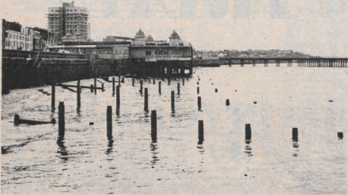
Promenade, pavilion and pier
