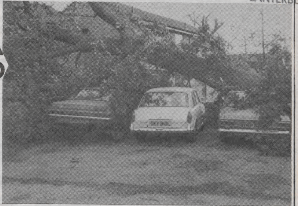
Cars which were crushed in Bishopden court Parkwood
