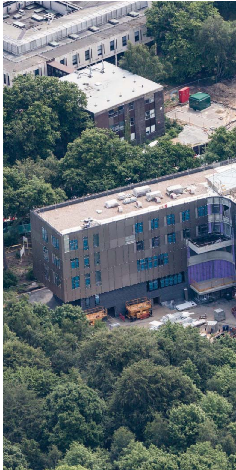
Figure 98: The Sibson Building in Brotherhood Wood nearing completion in 2017. Brotherhood Square is gradually taking shape in the top of the photograph
