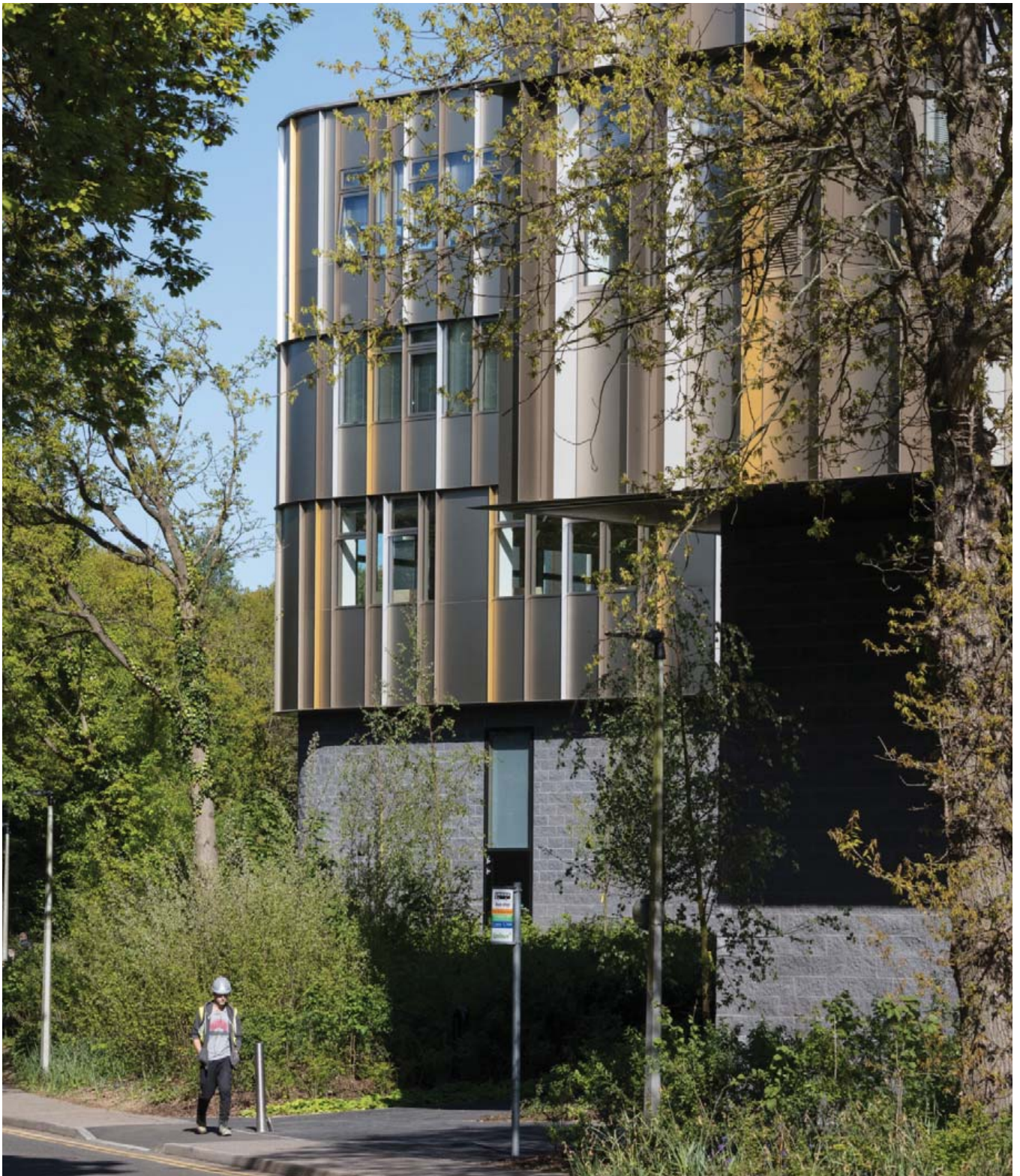
Figure 96: The Sibson Building in Brotherhood Wood; an example of a building designed to sit comfortably into the landscape
