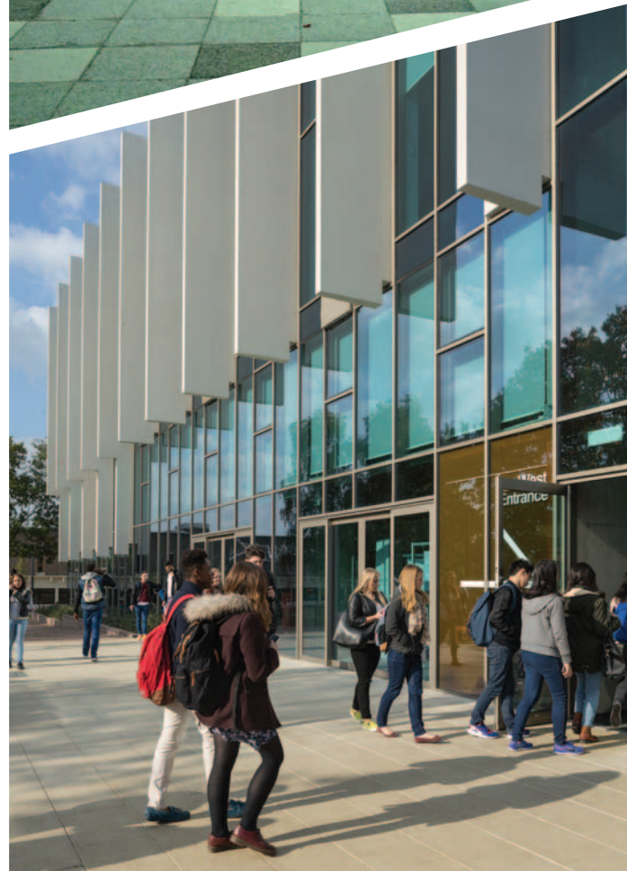
Top: Jarman School of Arts Building Bottom: Extension to the Templeman Library
